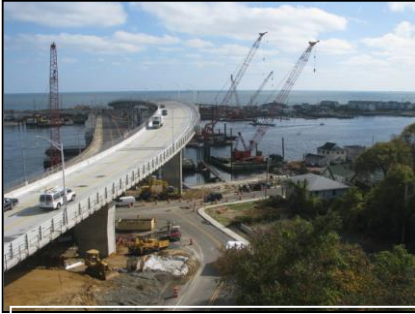
NJDOT Route 36 Highlands Bridge
