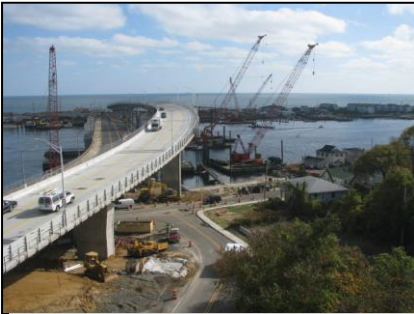
NJDOT Route 36 Highlands Bridge
