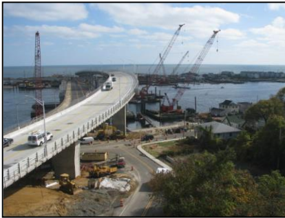
NJDOT Route 36 Highlands Bridge
