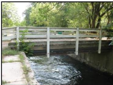
Delaware & Raritan Canal Dredging
