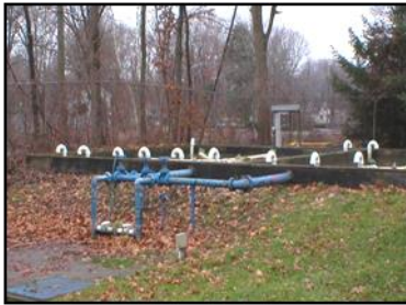
Sewage Treatment Plant Upgrade
