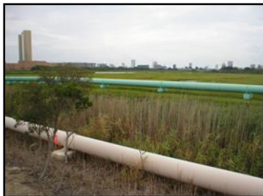
ACUA Reclaimed Water Line Crossing
