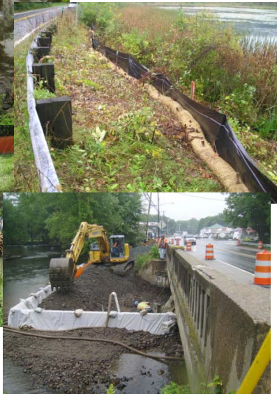
Exclusion fencing for bog and wood turtles, Route 94 Blair Creek, Blirstown, NJ
